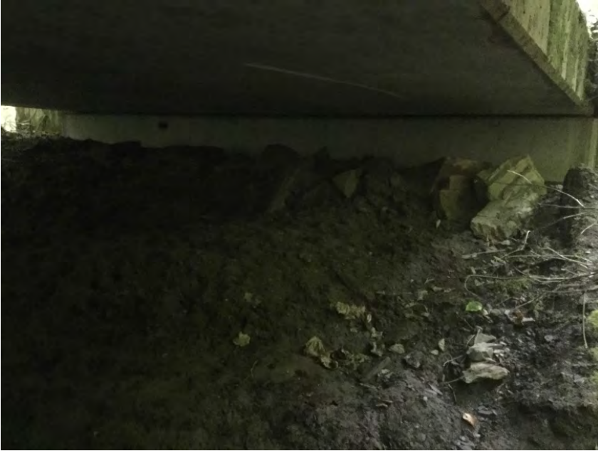
Right Bank Abutment when facing downstream
