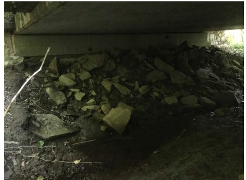
Left Bank Abutment when facing downstream
